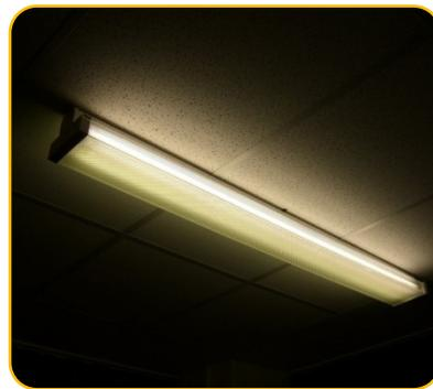
*As PCB-containing light ballasts age, the chance that they will leak or catch fire increases.*
